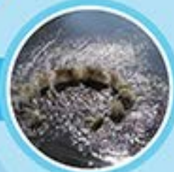
Wipes can combine with fats and grease in the pipe to form "Fatbergs" and are the primary causes of overflows from the manholes.
