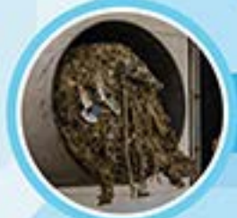
Wipes can cause breakdown of pumps in pump stations.
